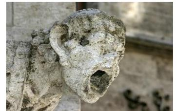
Abb. 5: A gargoyle that has been damaged by acid rain [1]
